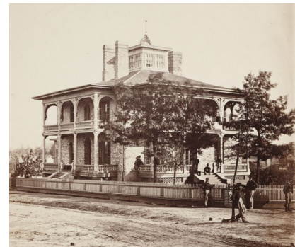
Calico House on SE corner of Collins St and Wheat St.
