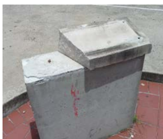
Left: Broken concrete base.
