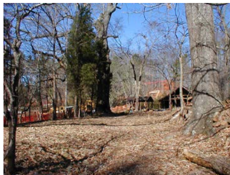
January 2003: Looking N along Wallis House driveway. Signal Hill is beyond construction in middle distance.
