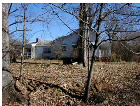
January 2003: Looking E towards house.
