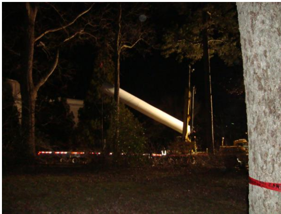
Scroll 1 being lowered onto flatbed truck, evening of 9 February.
