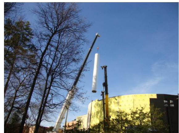
Scroll 2 being lowered into new building, afternoon of 10 February.
