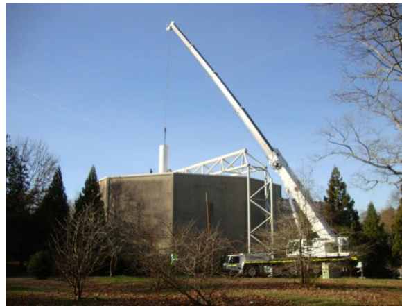
Scroll 2 being lifted from Grant Park building, morning of 10 February.
