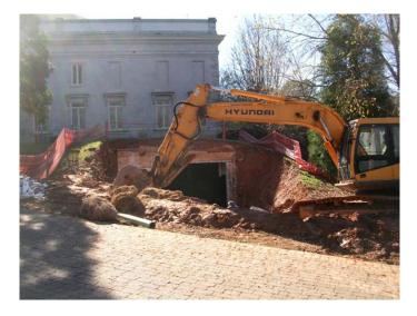
Left top: Underground north wall of building removed. Buried utility lines prevented clearing of a flat pathway. Consequently, Texas and its tender were pulled upslope for the last several yards before being lifted onto trucks.
