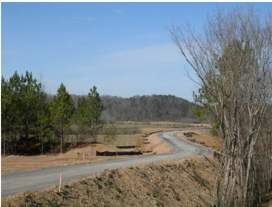
Photo looking north from future park entrance along access road.
