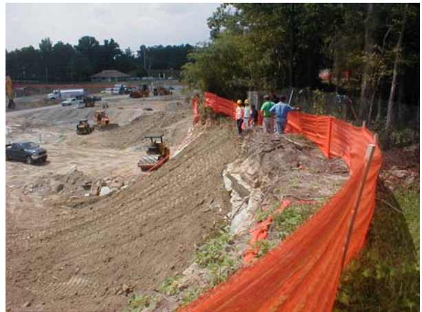
The initial repairs on afternoon of 28 August.
