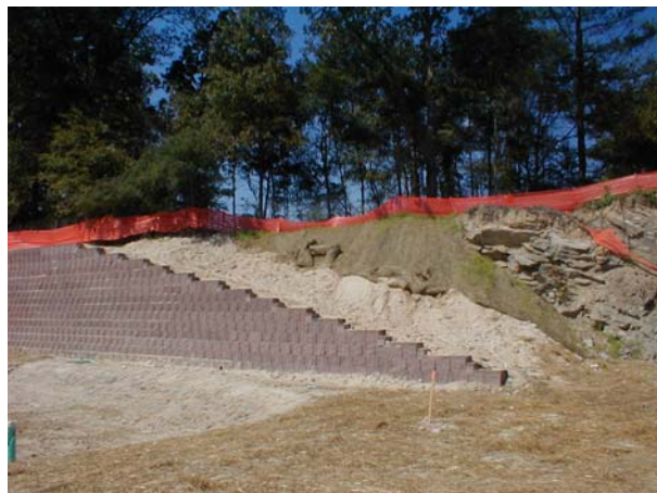
Retaining wall and initial fill on 27 September.
