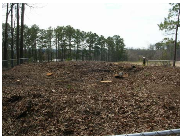
Smyrna Shoupade cleared of trees. The land in front of the Shoupade will be soccer fields.
